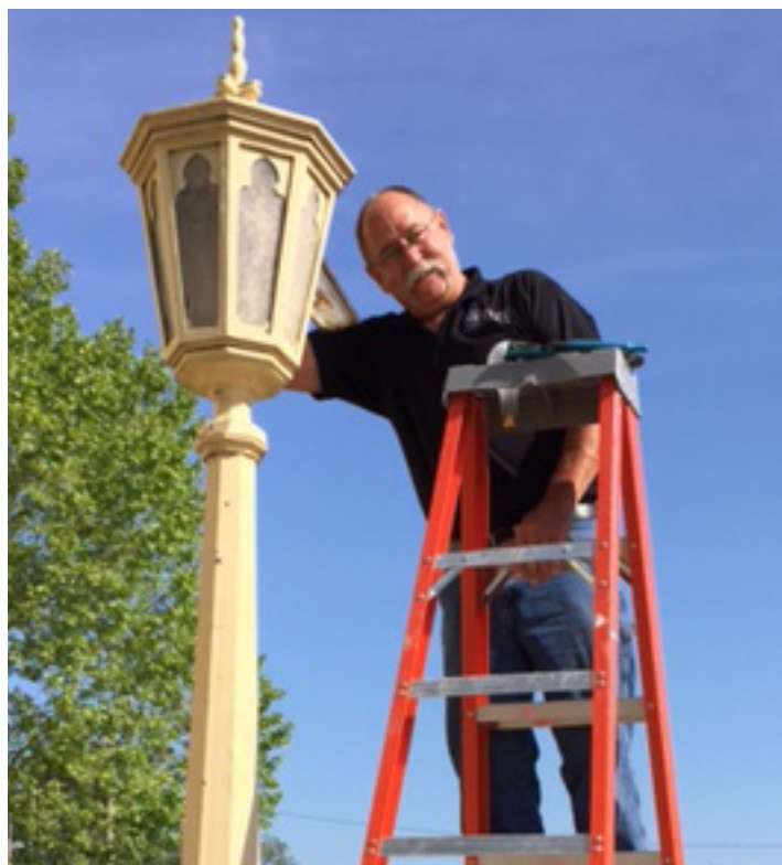
Mark Menges repairs the wiring on one of the lamp posts outside the front of the church.
